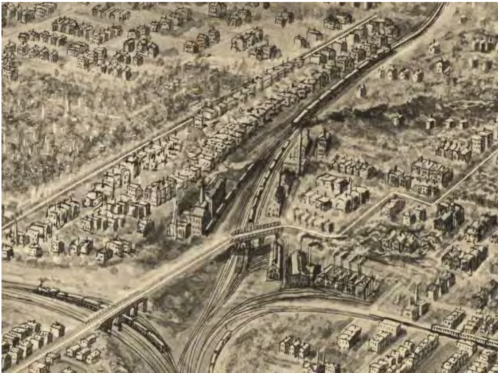
This 1906 panorama shows workers housing sprouting up on the western edge of the valley, and industrial buildings in the valley floor—likely related to the railroads. St. Paul, Minn, by Robert Saint. (Library of Congress)
